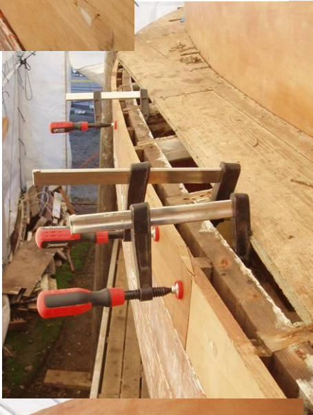
Fitting the new sheer strake
