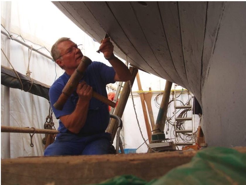
Re-caulking the seams begins - about 550 feet to do!
