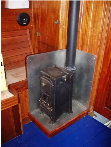
The refurbished stove with new flue pipe installed in the main cabin. The floor isn't really this blue!
